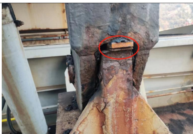
End hinge was worn out heavily
