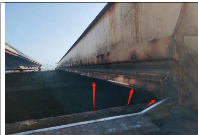
the condition of drain channel
