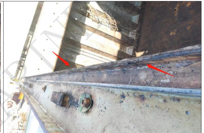
Drain gutter was rusty
