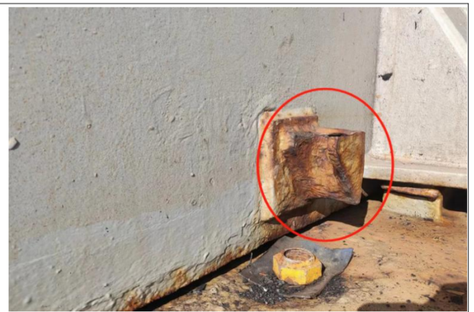
Drain gutter was rusty
