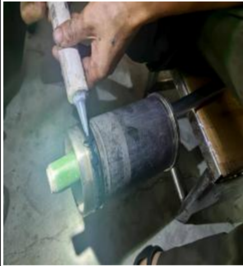
Coating the sealant for liner.
