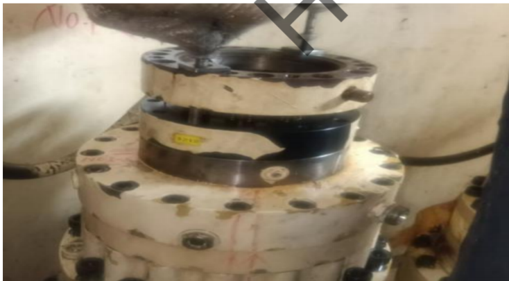
Install slewing brake
