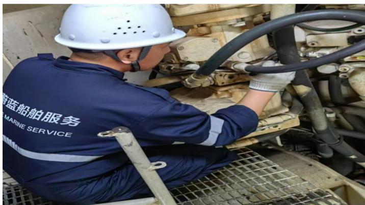
Made marks before dismantle the pumps to avoid wrong matching
