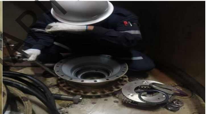
overhaul the gearboxes
