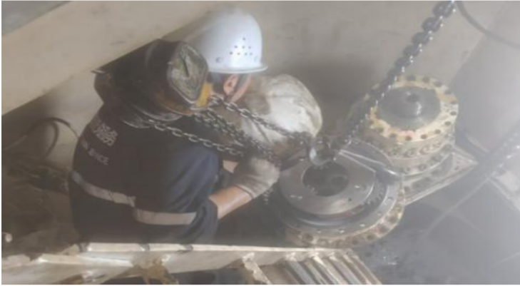
overhaul the gearboxes
