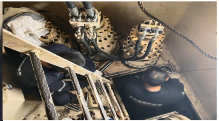
Renew the slewing unit rubber hoses
