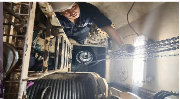
overhaul the gearboxes
