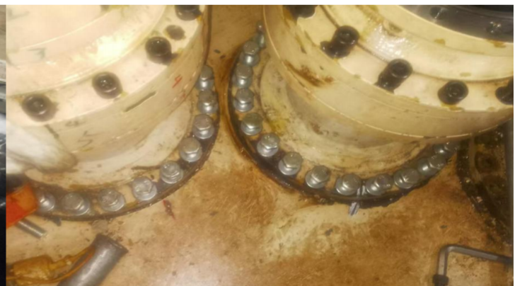
overhaul the gearboxes
