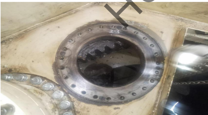
overhaul the gearboxes
