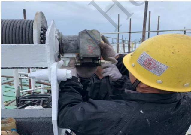
Limit switches adjustment and final commissioning
