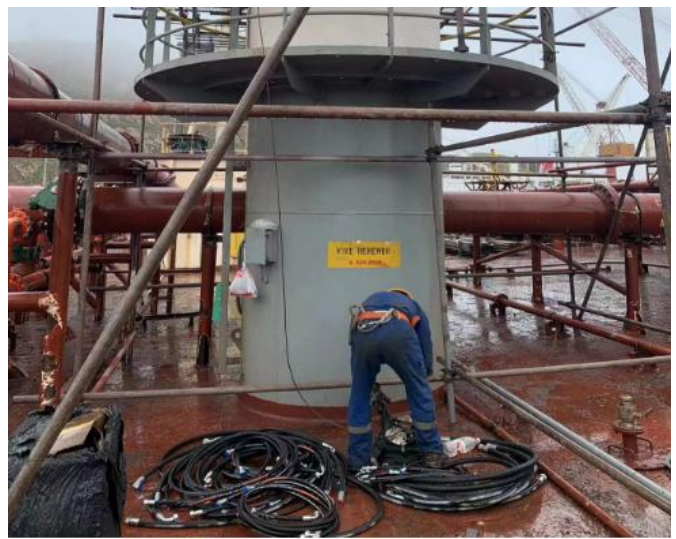
Install the new spare control blocks, keep overhauled old control blocks on board as spare
