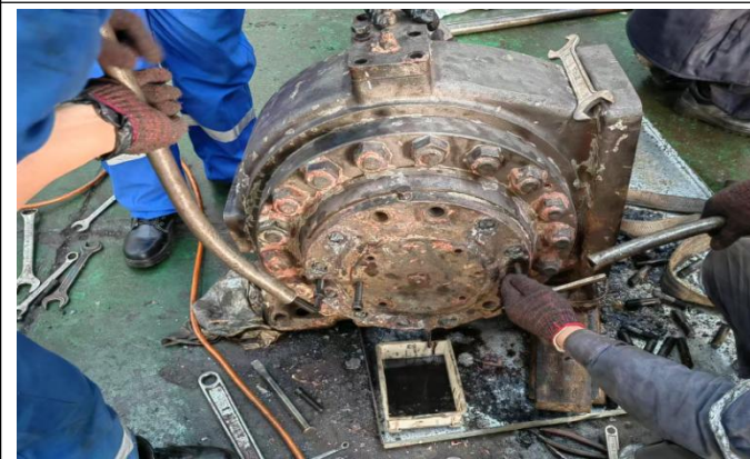
Disassemble the hydraulic motors
