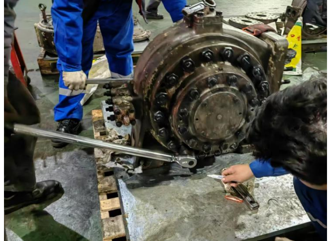
Tight the hydraulic motor side cover by torque wrench
