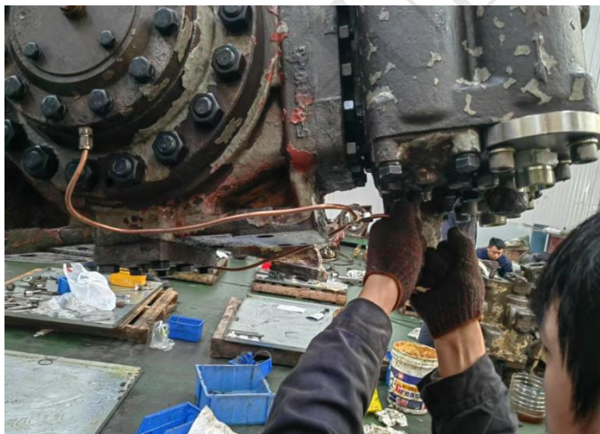
Renew copper pipes and fittings
